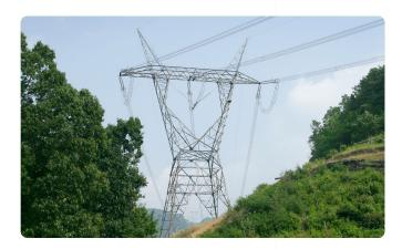
In addition to the wires carrying the electricity, one or two ground wires protect the tower from lightning strikes. Before electricity can travel from the transmission system and be delivered to your home, it has to make a stop at a substation.
